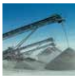
GRAVEL AND CONCRETE PLANTS
